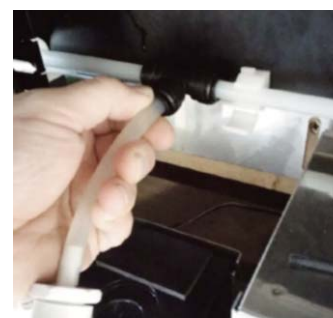
5. Disconnect pump from tee
